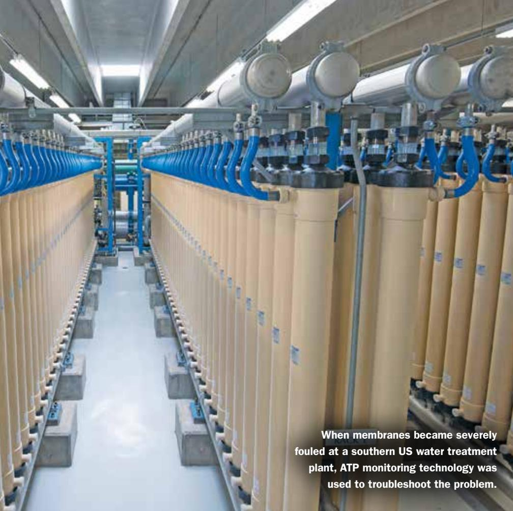
When membranes became severely fouled at a southern US water treatment plant, ATP monitoring technology was used to troubleshoot the problem.
